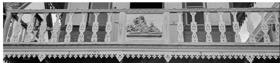
While at Cobham Hall, perhaps because some were rotten, the balusters edging the balcony were thinned out. Our scheme would see new (matching) balusters reinstated alongside the remaining originals, overcoming the health and safety issue and restoring the original close-set look.
