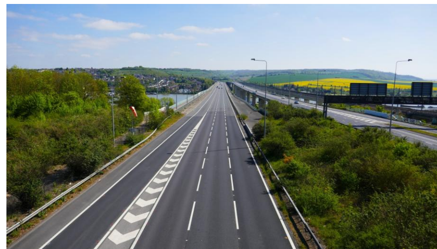
A closer view of Rochester M2 motorway bridge, Saturday 25 April 2020
