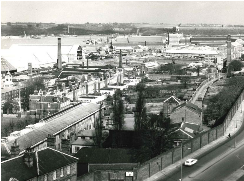
Chatham Dockyard taken on 18 March 1970 from nearby flats and published in the Evening Post; Medway Archives Centre, ref: CHA/AN/DYD/AV/7.
