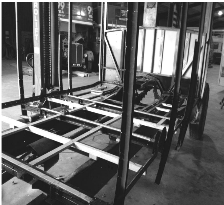
The body structure reconstruction under way, early 2014. Photograph, R. J. Bourne.
