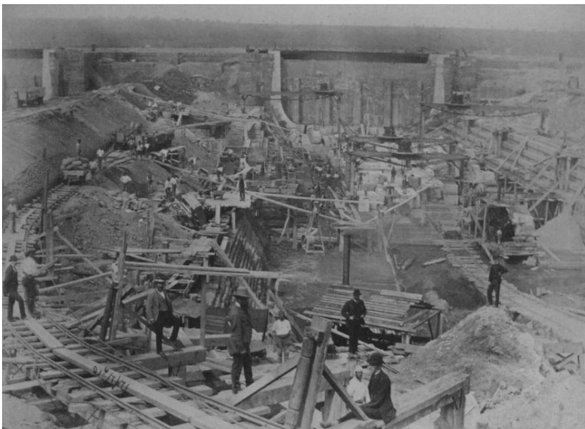
Building Dock no. 8; note the caisson is already in place as part of the basin.
