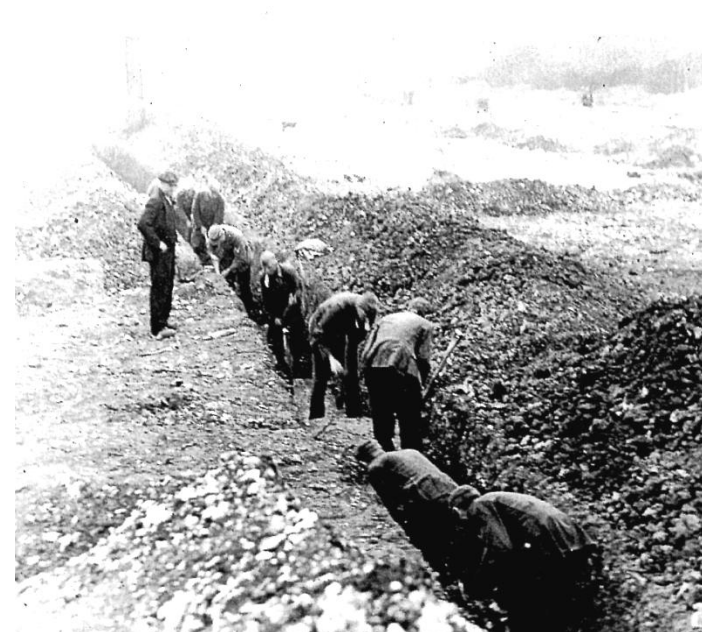
PoWs digging prefab drains.
