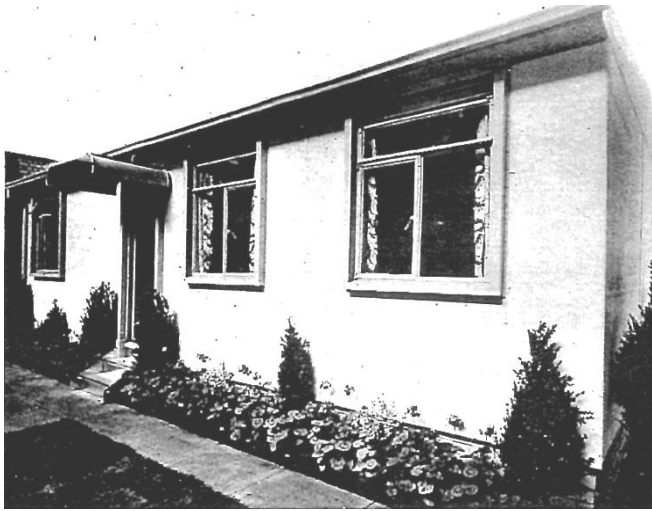
An exterior view of a typical prefab; Illustrated London News, 1945.
