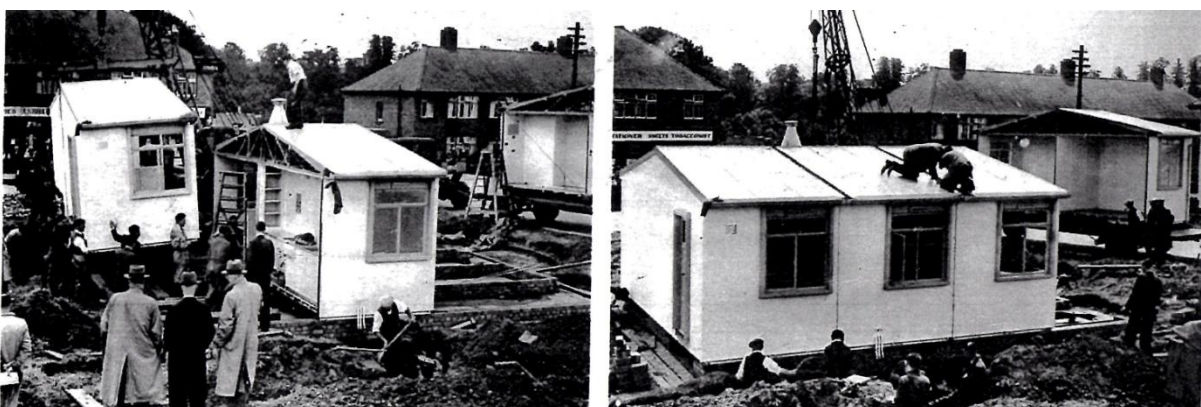
The final stages of prefab erection, Illustrated London News, 1945.
