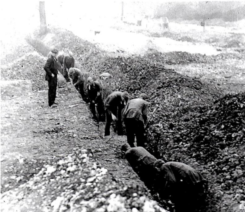
PoWs digging prefab drains.
