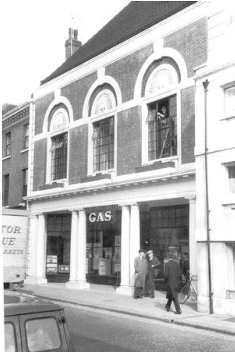
The Gas Board showrooms photographed in 1967, number 95, on the north side of Rochester High Street (west), previously numbered 58. J. L. Edwards, Mayor of Rochester, lived here in 1873. Medway Images, ref. C050772633; Medway Archives and Local Studies Centre.
