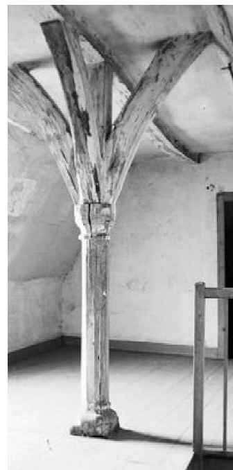
A roof truss from the hospital, salvaged and photographed here in Eastgate House; The Medway Archives and Local Studies Centre.
