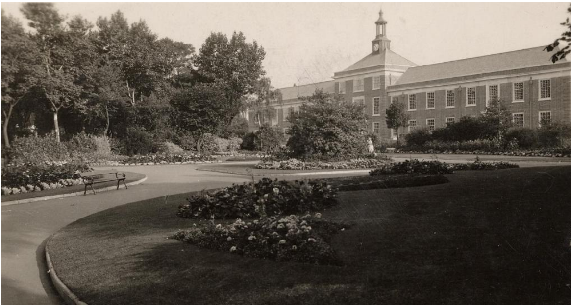
The Municipal Buildings, Gillingham; postcard original from the Medway Archives and Local Studies centre Couchman Collection; DE402/21/40
